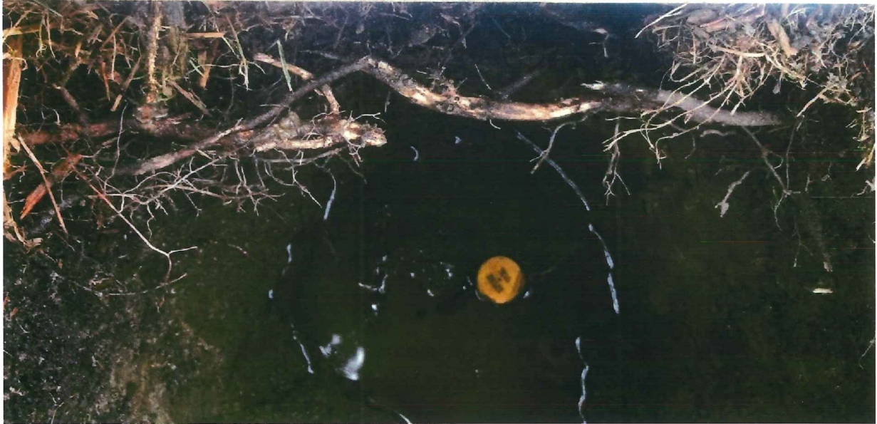
BEFORE FI1/2"x30" #38121 1.5' below ground, remains of Mon fnd. (04/16/2014)
